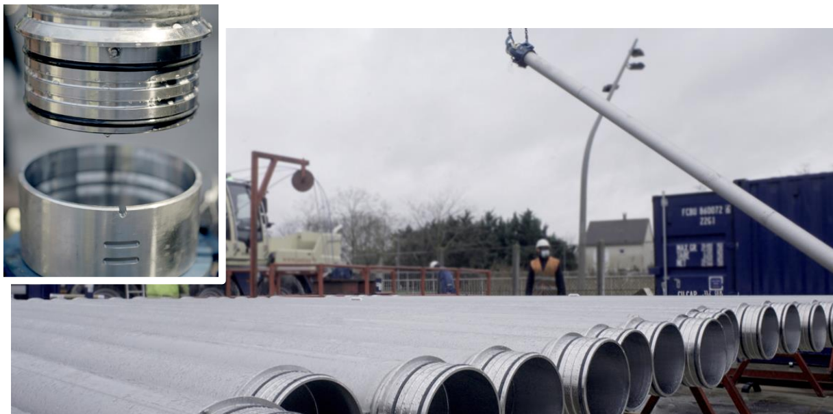
Figure 2 – Installation of DN175 diameter riser pipe
