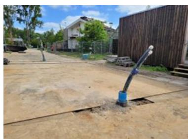
These two bore hole heat exchangers were the first two installations constructed with Directional Steel Shot Drilling, retrofitted on a Remborg 15 tons Conrad drilling machine. The drilling was steered and each BHE constructed within 4 days.
