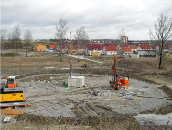
Fig. 6: Installation of the 80 BHEs at the BTES in Crailsheim, Germany [9]
